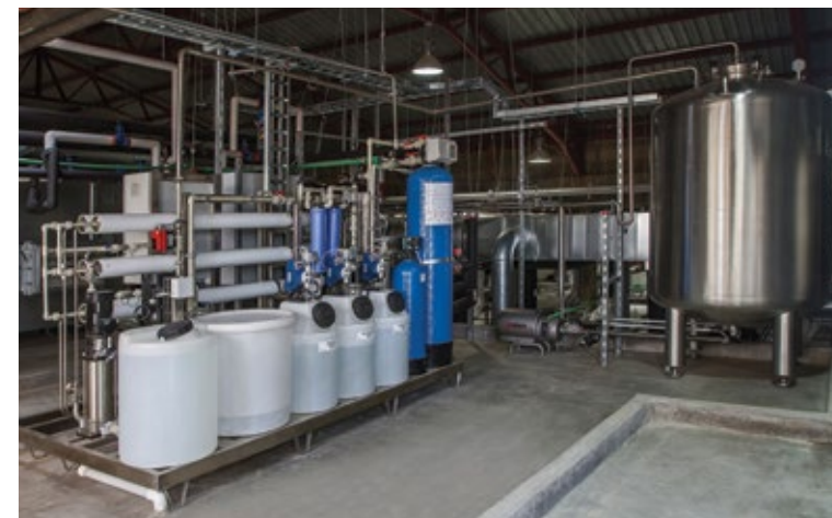
Water pre-treatment and generation of purified water, including loop for water distribution and storage tank
