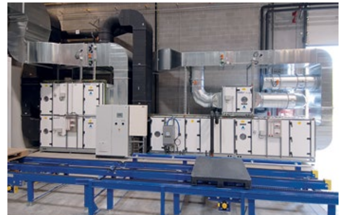
Upper image: Complete installation of air makeup and handling units for a laminar flow of 26.600 m 3 /h.
