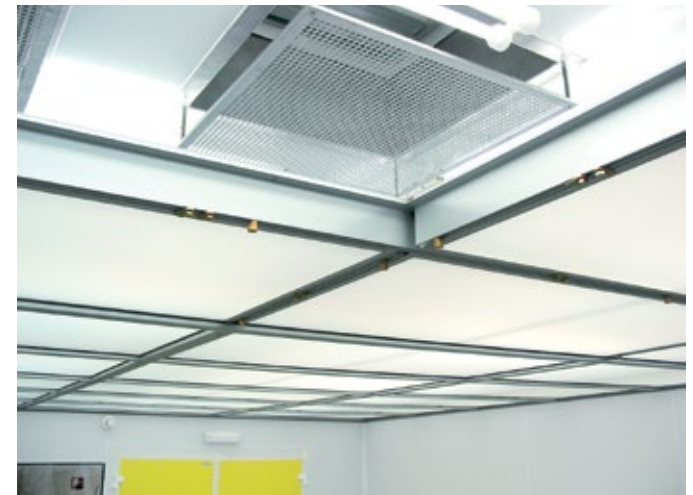
Laminar flow installed with a dismantled diffuser membrane.
