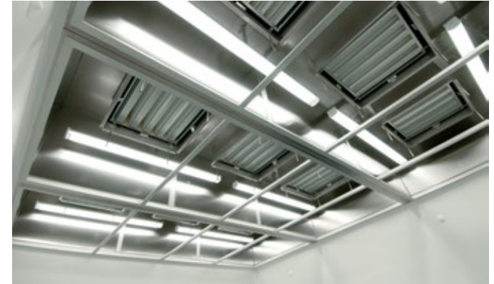
Detail of the interior part of a laminar flow module: HEPA filters and lights before placing diffuser membrane.
